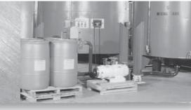
The RL9000 TWM tank weigh module's **I** stainless steel construction provides accurate weighing technology for hostile environment applications. Its low profile configuration maximizes space and its all-in-one construction minimizes installation time. Furthermore, the RL9000 TWM will accurately weigh even if the base is off level by as much as 3°.
